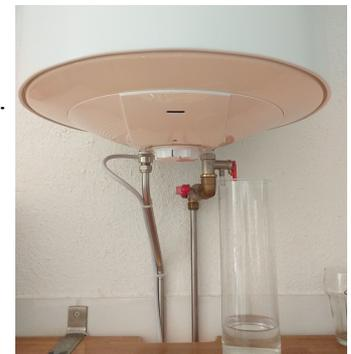
The, during the heating, expanding water is collected in the vase for recycling and as boiler-use indication.
